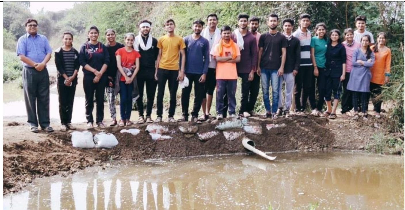
Construction of ENB for increasing groundwater recharge by the NSS students in the NSS Camp of Our college 2019-20
